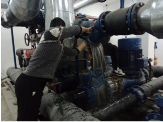
2#交换站供暖除污器清堵
